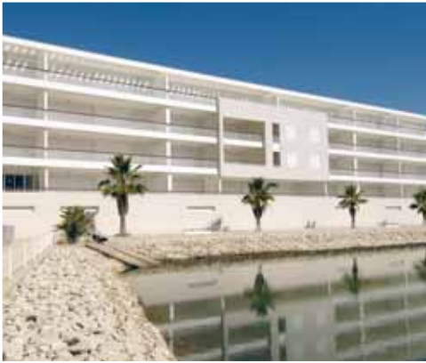
Edifício Pedro Álvares Cabral, Marina de Lagos, Algarve Pedro Álvares Cabral Building, Marina de Lagos, Algarve
